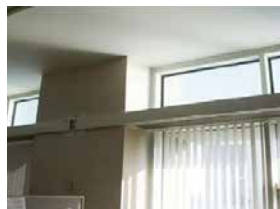
3M Daylight Redirecting Film (Daylighting Zone)
