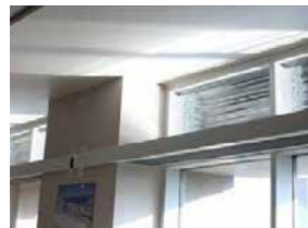
Daylight Redirecting Blinds (Daylighting Zone)
